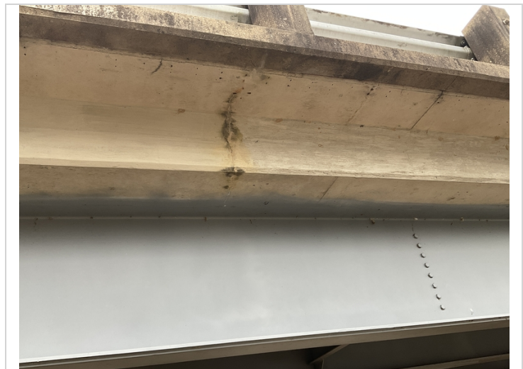
03/2022... cracking on overhangs various locations
