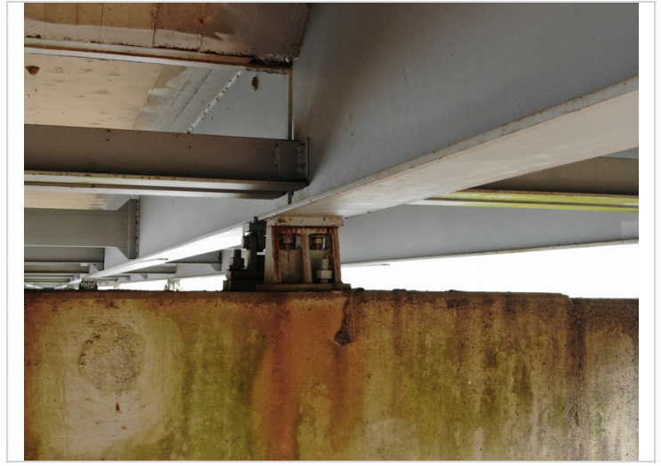
CS2 Corrosion Bearing Bent 6
