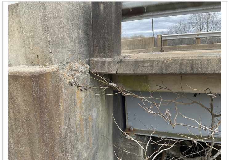
03/2022... spall and crack Rt side beginning of bridge
