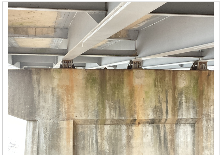
03/2022... anchor bolts are backing out or not tightened at various locations
