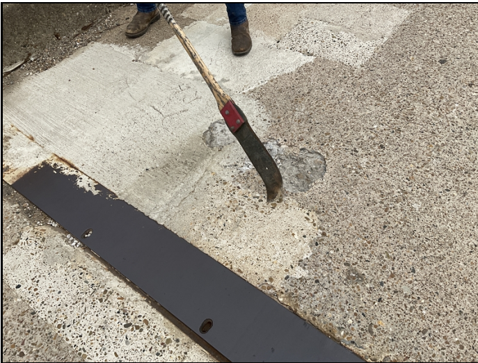
03/2022... LT side span 6 existing patch spalling
