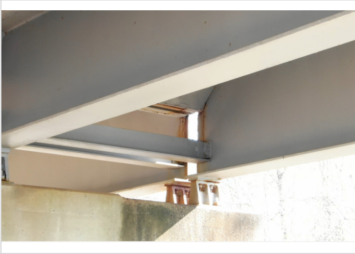
CS2 Corrosion Bent 7
