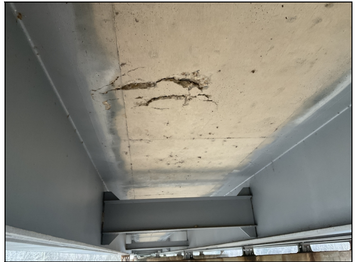
03/2022... Rt side last span delam
