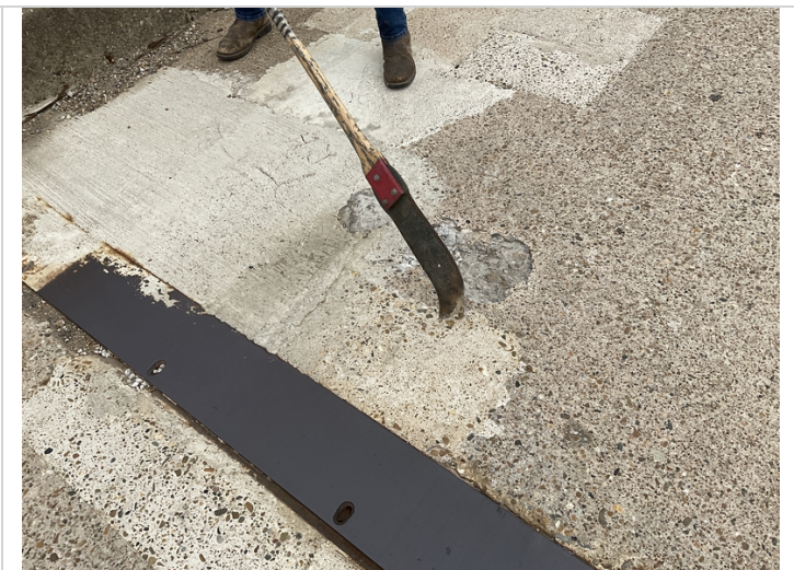
03/2022... LT side span 6 existing patch spalling
