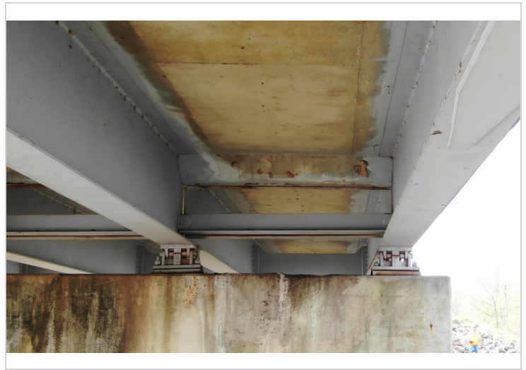
CS2 Corrosion Bearing Bent 3
