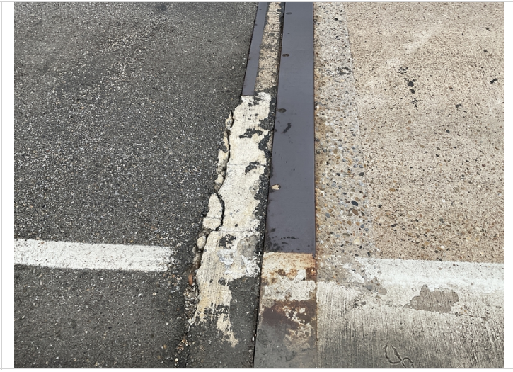
03/2022... end of bridge approach cracked and damaged
