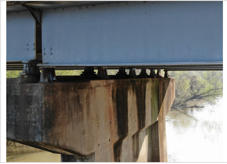
Cracking Bent 7 Cap
