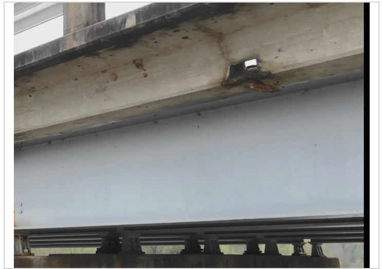
Spall - Exposed Bar
