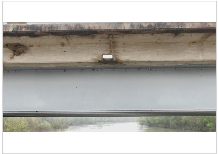
Crack/Delam at gutter
