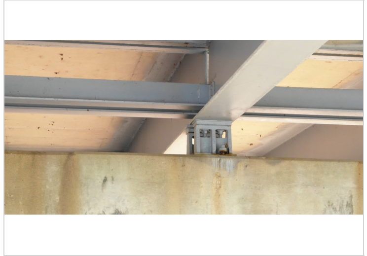
CS3 Corrosion Bearing Bent 9
