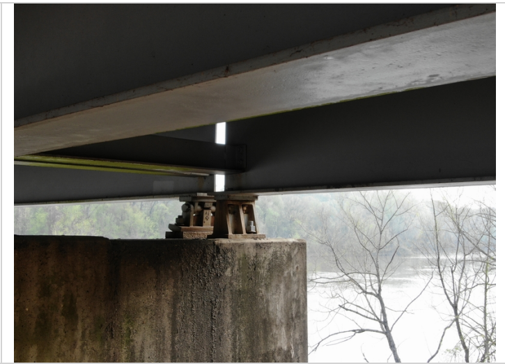
Bearing Position at 65 Degrees
