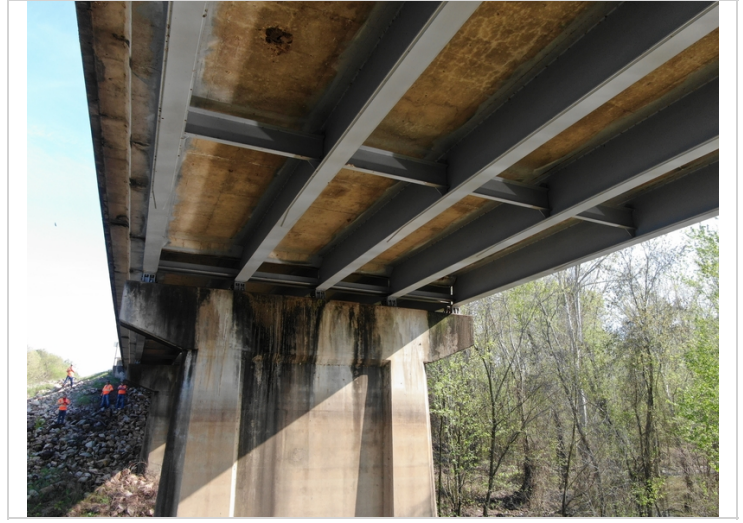
Span 7 Deck crack with Efflorescence
