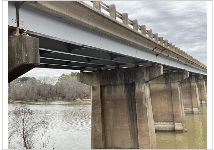
03/2022... steel beams typical all spans
