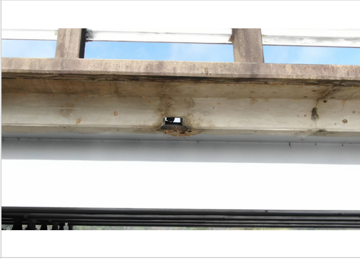
Exposed Bar Downstream Span 3
